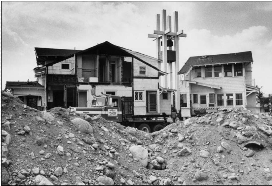
Grove House split in two
